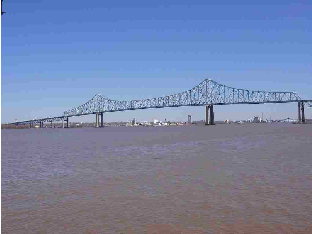
Figure 5.2 Overview of the Commodore Barry Bridge (From Wikipedia, http://en.wikipedia.org/wiki/Commodore_Barry_Bridge )
